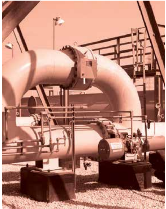
Buckling Pin Relief Valve installed as inline bypass to control valve on a gas flare system
