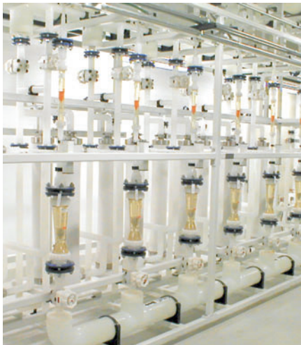
Basic supply of semiconductor factories, ultra pure water treatment
