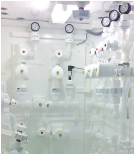
Chemical supply for wet processes
